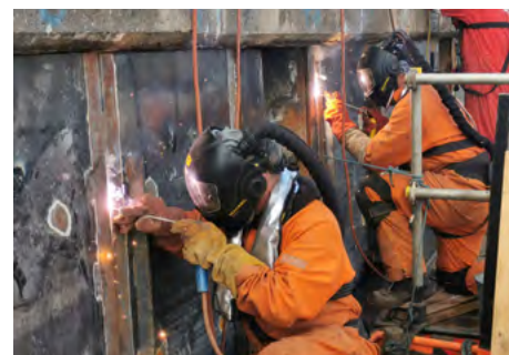
The £30 million NEC-procured coastal defence scheme included plating existing steel sheet piles
