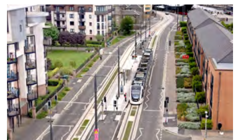
The final 4.7 km of line 1 was successfully delivered by two NEC4 ECC main contracts and completed in November 2023
