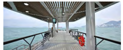
ECC Option X20 was used to incentivise the contractor to meet the client's safety objectives
