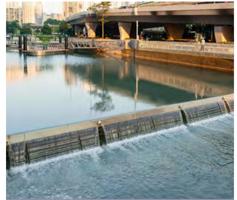
The NEC-procured restoration included an automatic 'smart gate' to optimise upstream water levels
