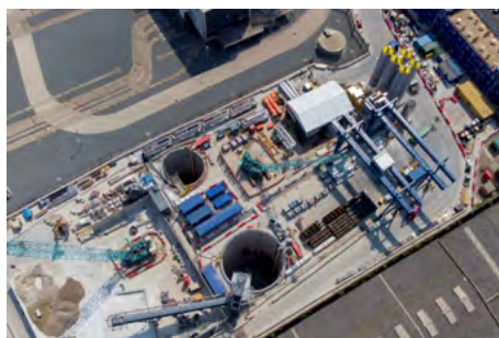
Five tunnel drives were undertaken from three drive sites using four tunnel boring machines
